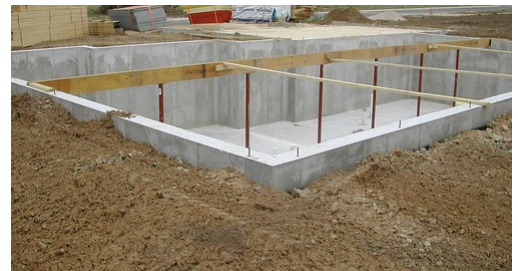
Example of a Permanent Foundation
